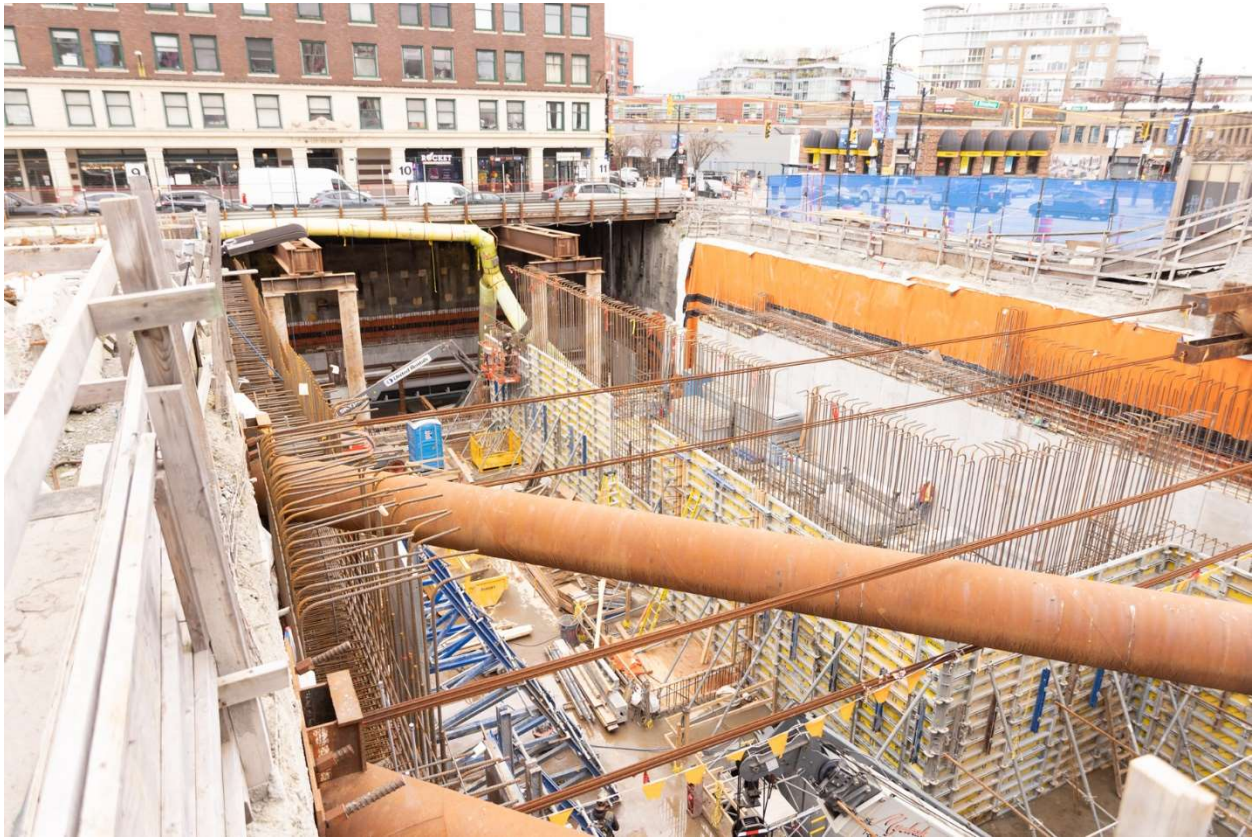
Figure 3: Mount Pleasant Station: Progressing with installation of rebar and concrete pours for the concourse-level walls in the headhouse.
