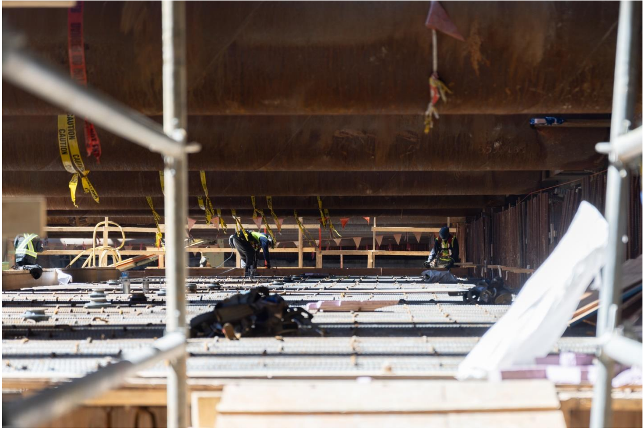
Figure 4: Broadway-City Hall Station: Progressing with construction of the concourse-level floor in the station.
