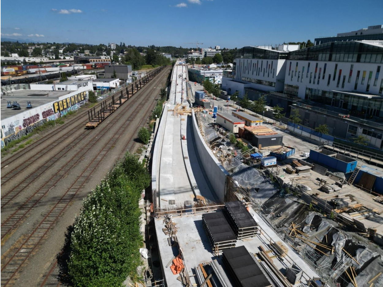
Figure 1: Elevated Guideway: Completion of the parapets at the abutment.
