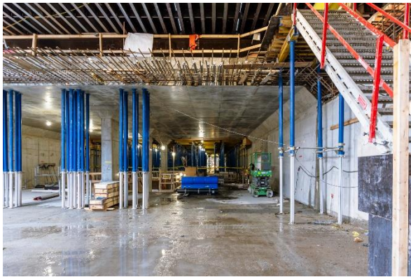
Figure 7: Arbutus Station: Progressing with construction of the underground station roof.
