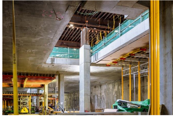
Figure 6: South Granville Station: Progressing with construction of the concourse-level floor.
