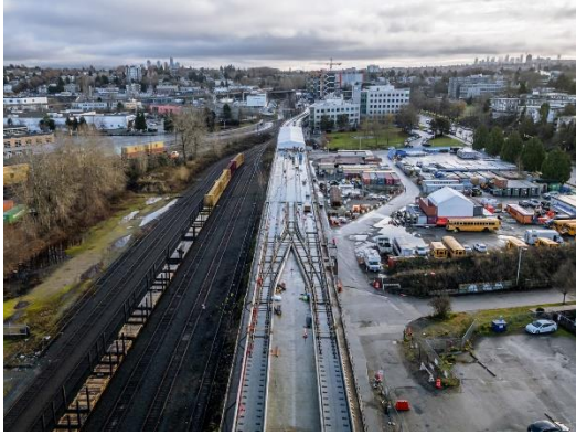
Figure 1: Elevated Guideway: Progressing with alignment of the pocket track switch.
