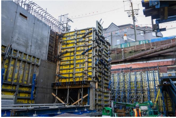
Figure 5: Oak-VGH Station: The interior walls in the headhouse being constructed.
